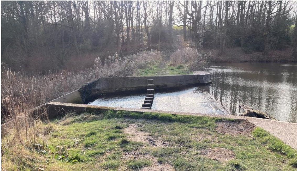
Picture 53 - The Weir
