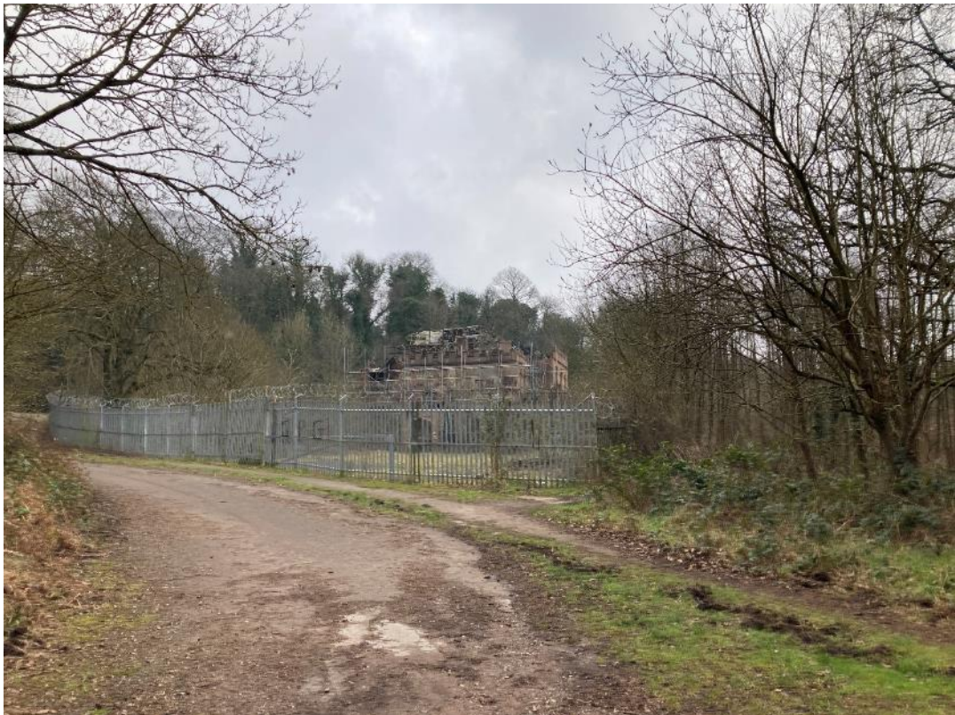
Picture 22 – Great Barr Hall from Sutton’s Drive
