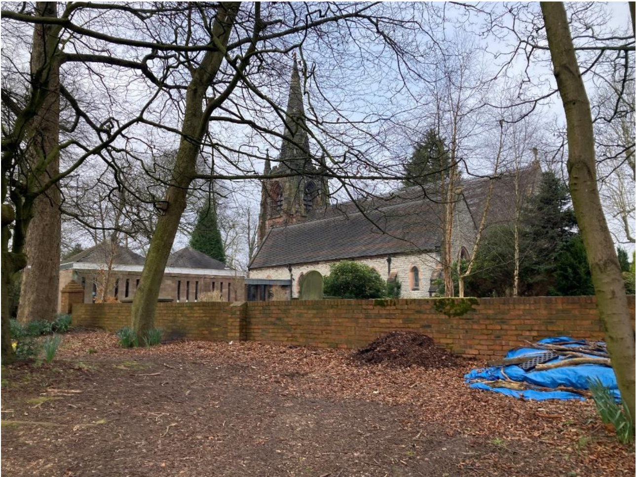
Picture 63 - Brick boundary wall to St Margaret's Church
