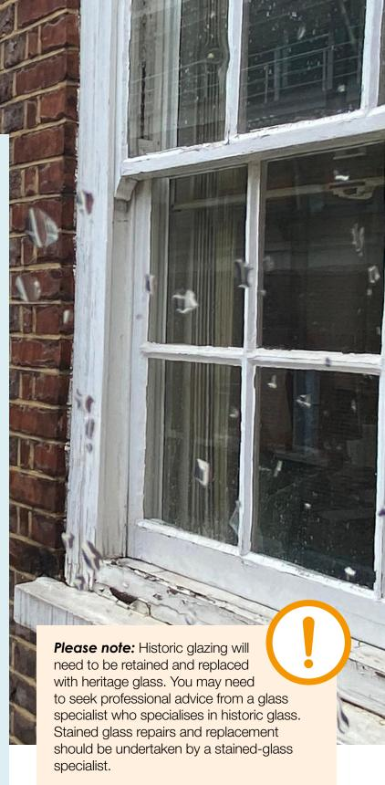
Works to cut out rotten timber and splicing in of new timber will need to be undertaken by a joiner/timber specialist, you are advised to seek professional advice from a joiner or a timber specialist.
