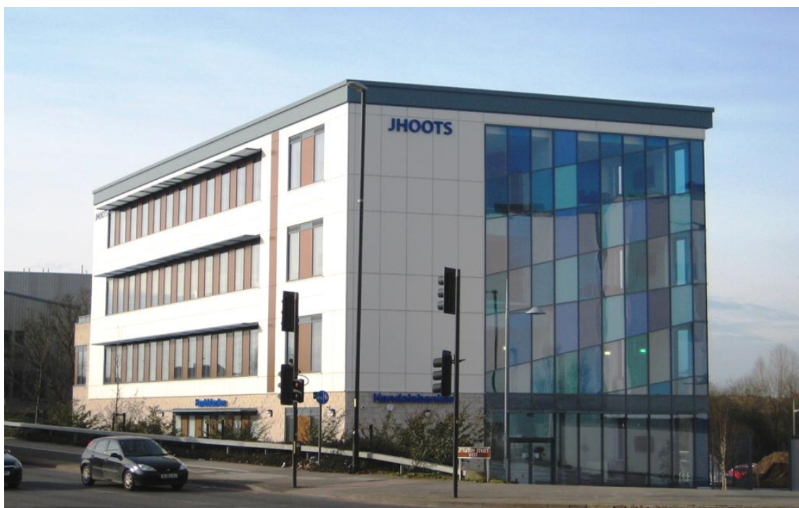
Figure 4.1 Jhoots Pharmacy headquarters, Littleton Street
