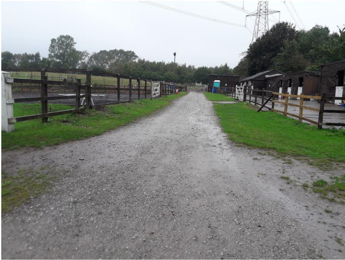
Photograph 5: Stable block and their associated hard standing. The surface arena can also be seen adjacent to the access road.
