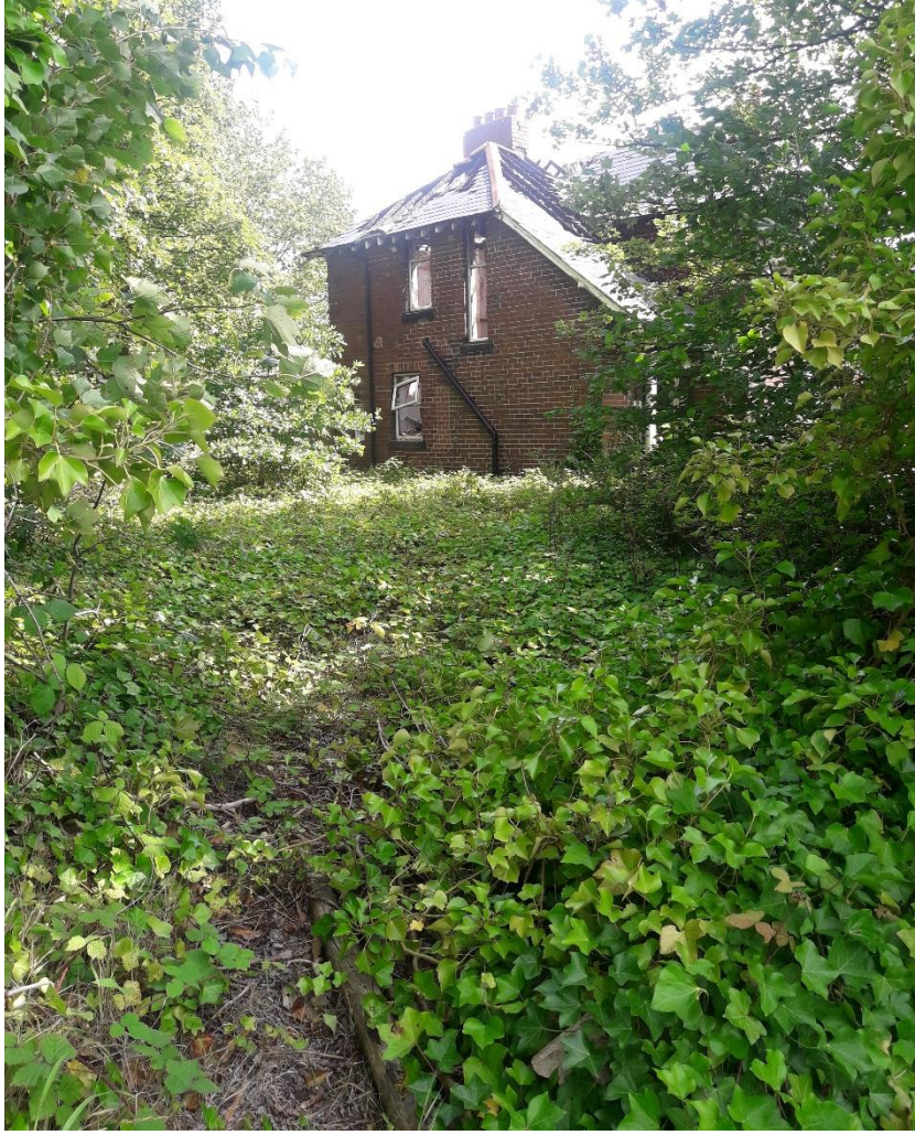
Photograph 3: House with fire damage surrounded by scattered trees.
