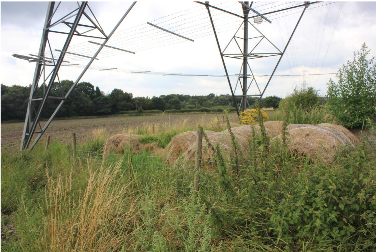
Photo 4: Area of tall ruderal vegetation under large metal electricity pylon, which also has a number of hay bales left underneath it.
