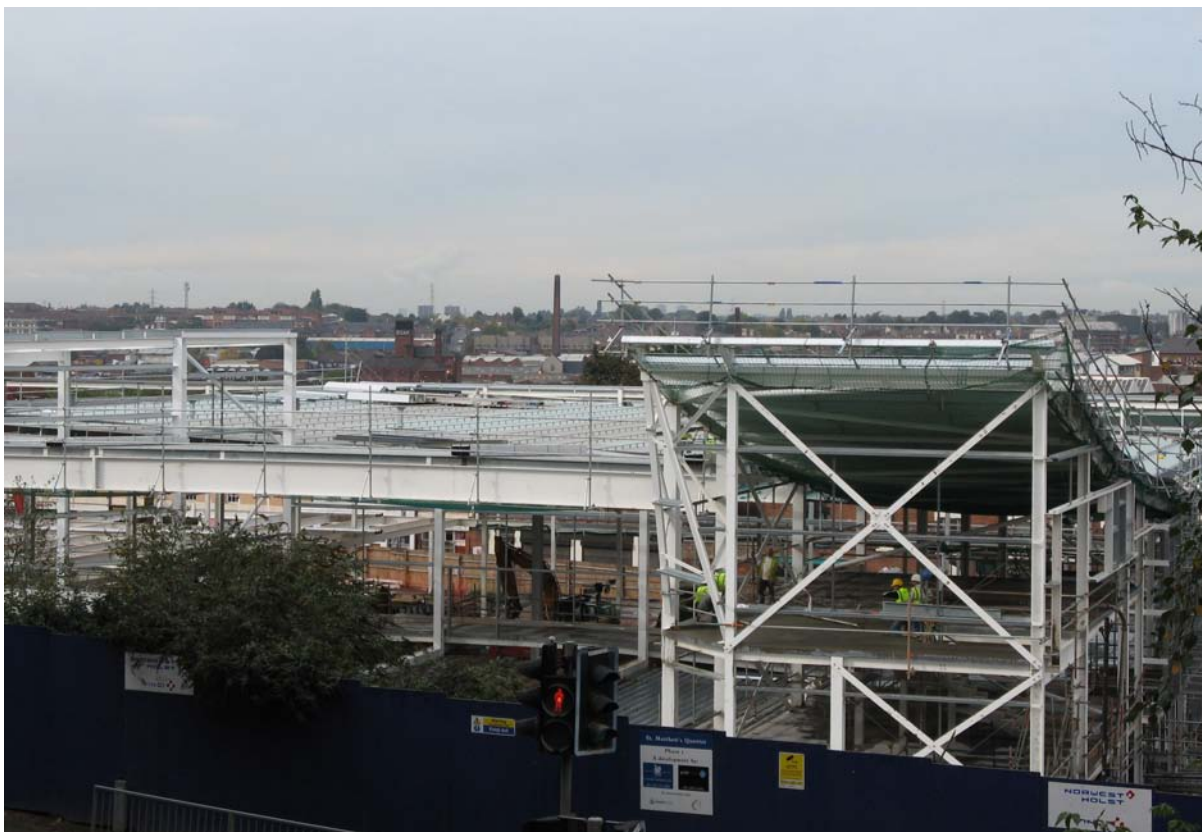
New foodstore under construction, Walsall
