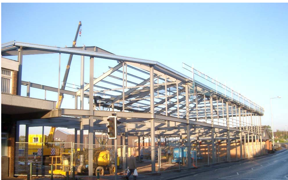
New Shops under construction, High Street, Brownhills
