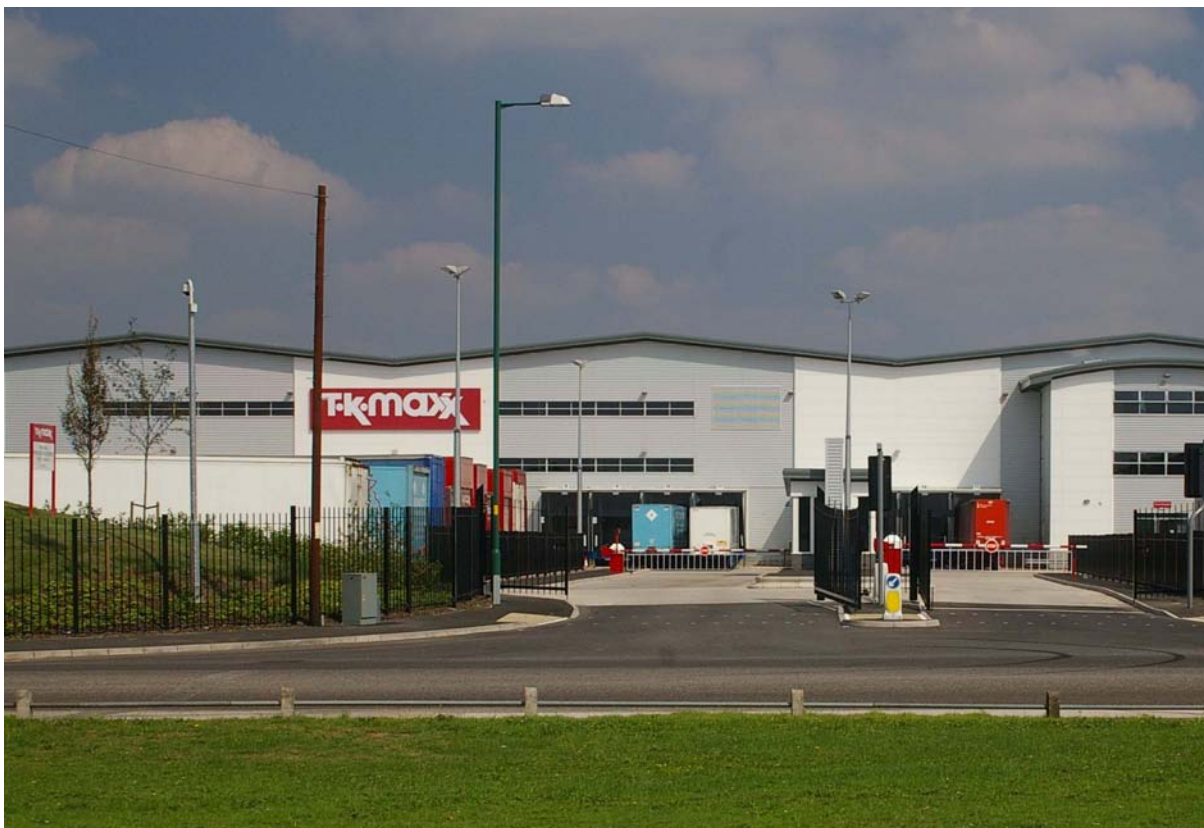
New warehouse for TK Maxx, Walsall
