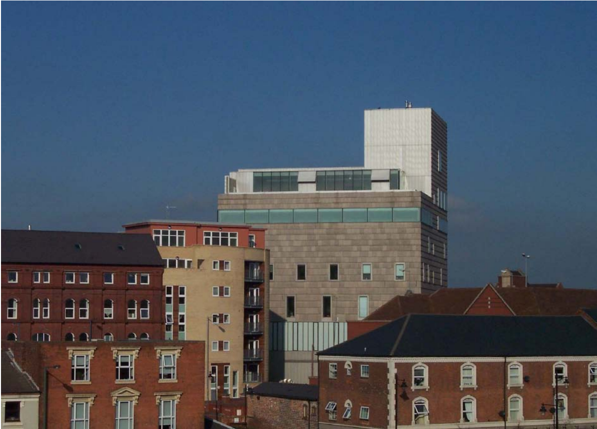
Residential and cultural uses in central Walsall
