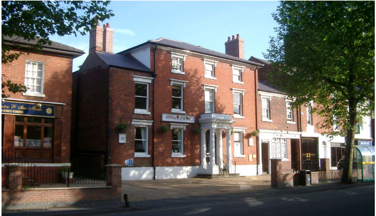
Refurbished office in Walsall
