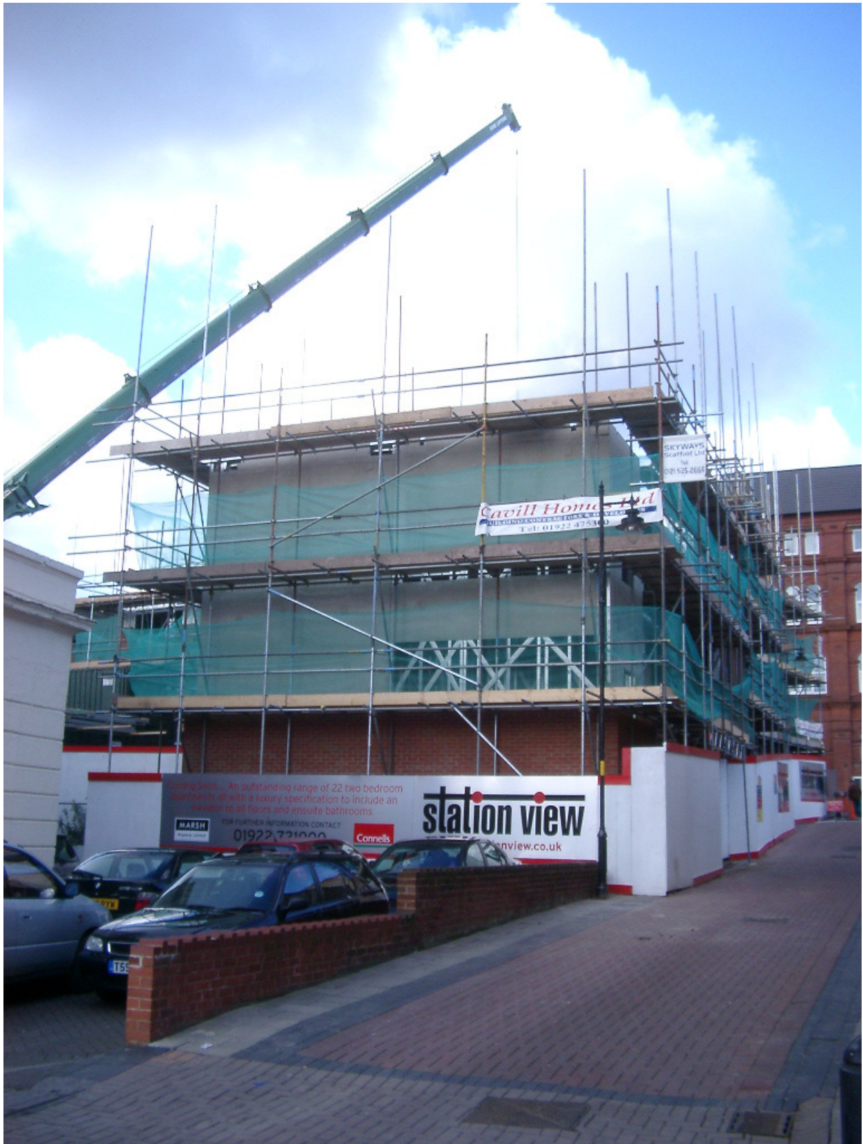
New apartments under construction close to Walsall's primary shopping area
