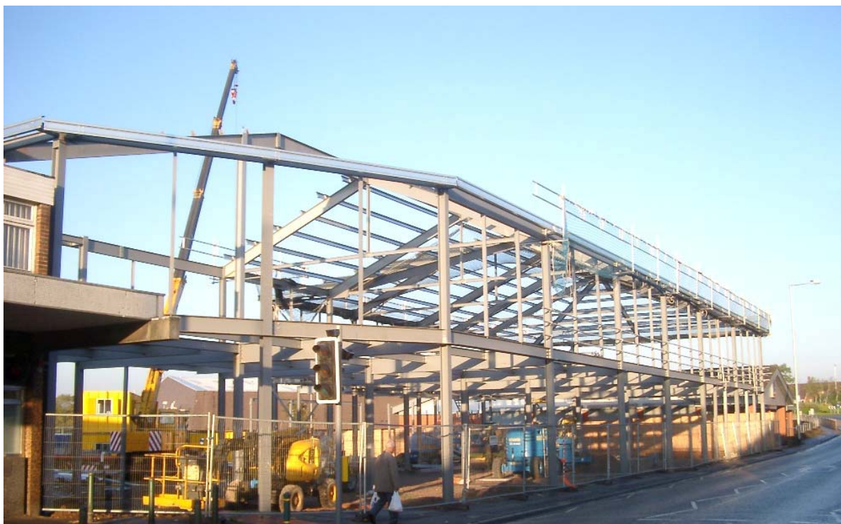
New Shops under construction, High Street, Brownhills
