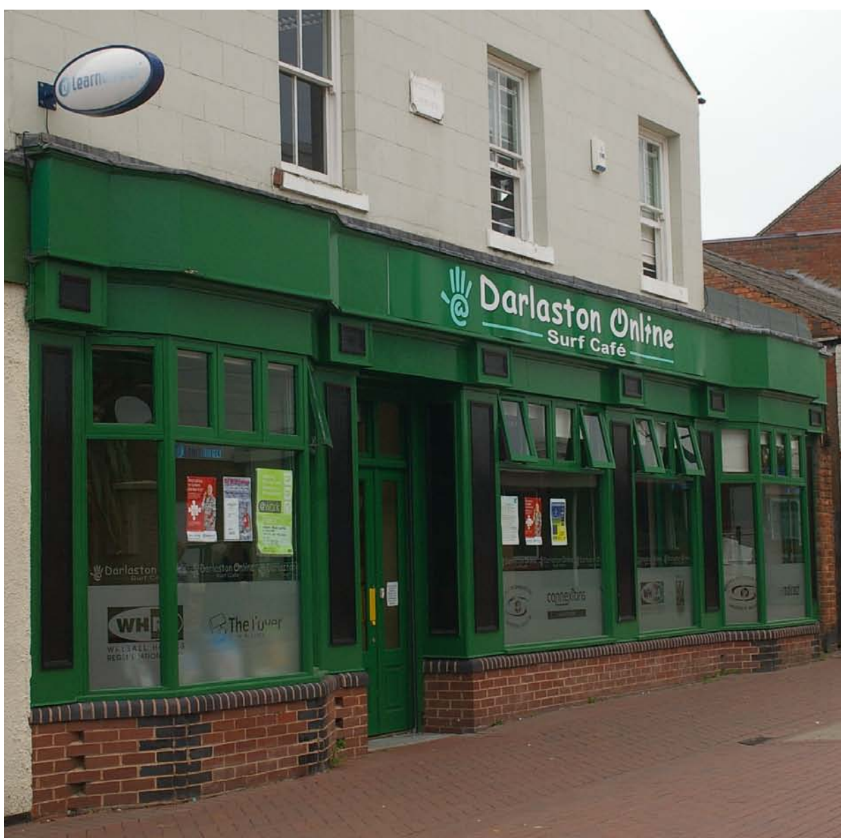
In Darlaston District Centre
