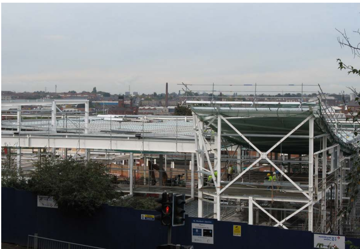
New foodstore under construction, Walsall
