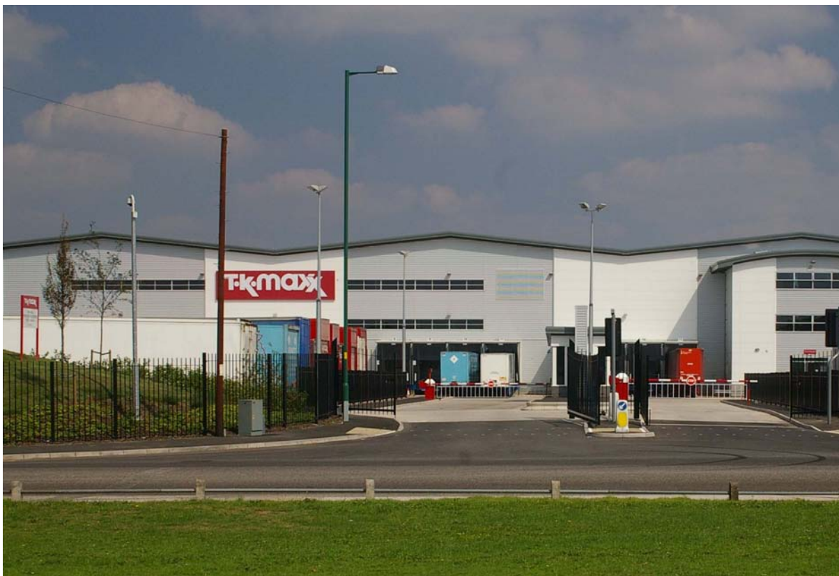
New warehouse for TK Maxx, Walsall
