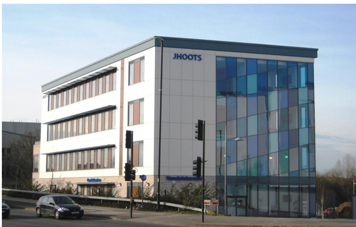
Figure 4.1 Jhoots Pharmacy headquarters, Littleton Street
