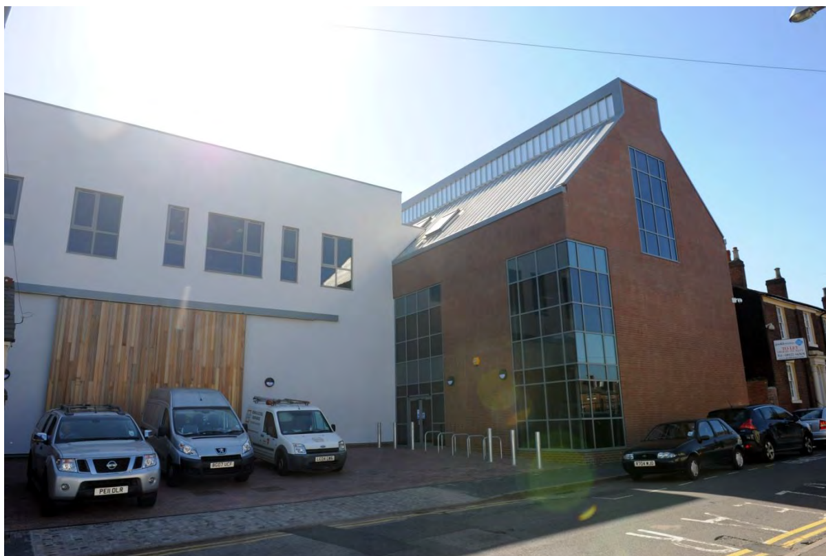
Figure 4.2 The Goldmine Centre, Lower Hall Lane
