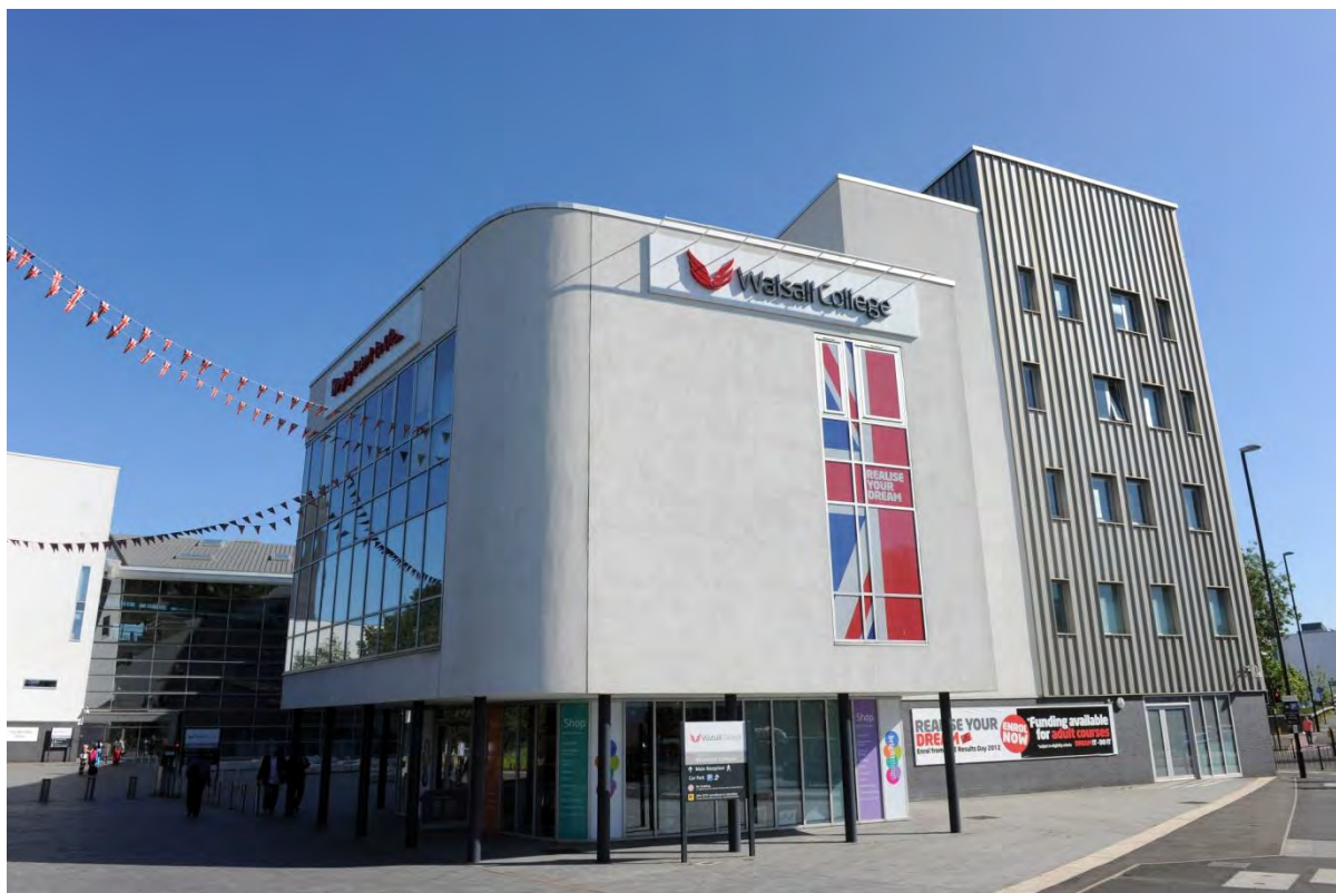
Figure 6.1 Walsall College, Littleton Street West
