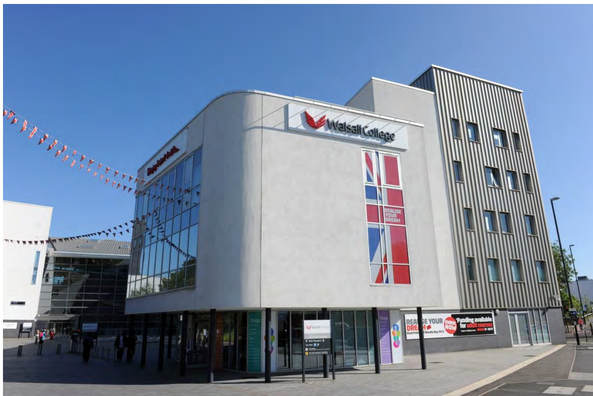
Figure 6.1 Walsall College, Littleton Street West
