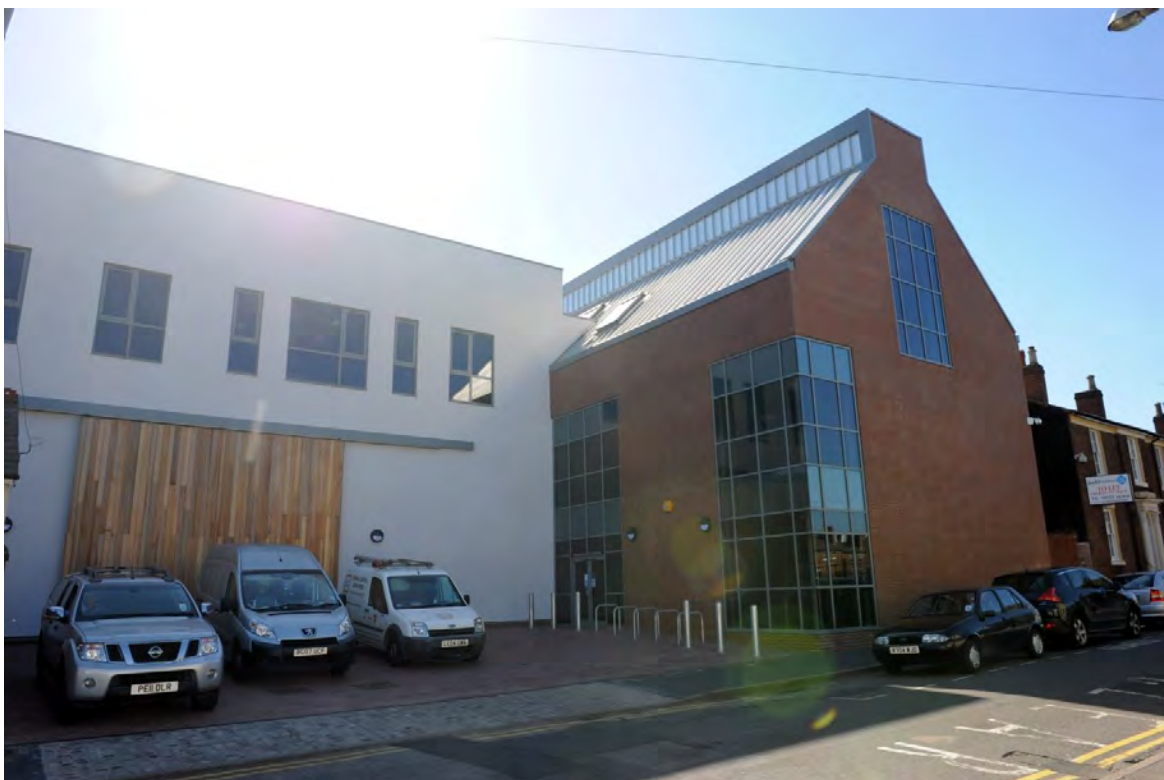
Figure 4.2 The Goldmine Centre, Lower Hall Lane
