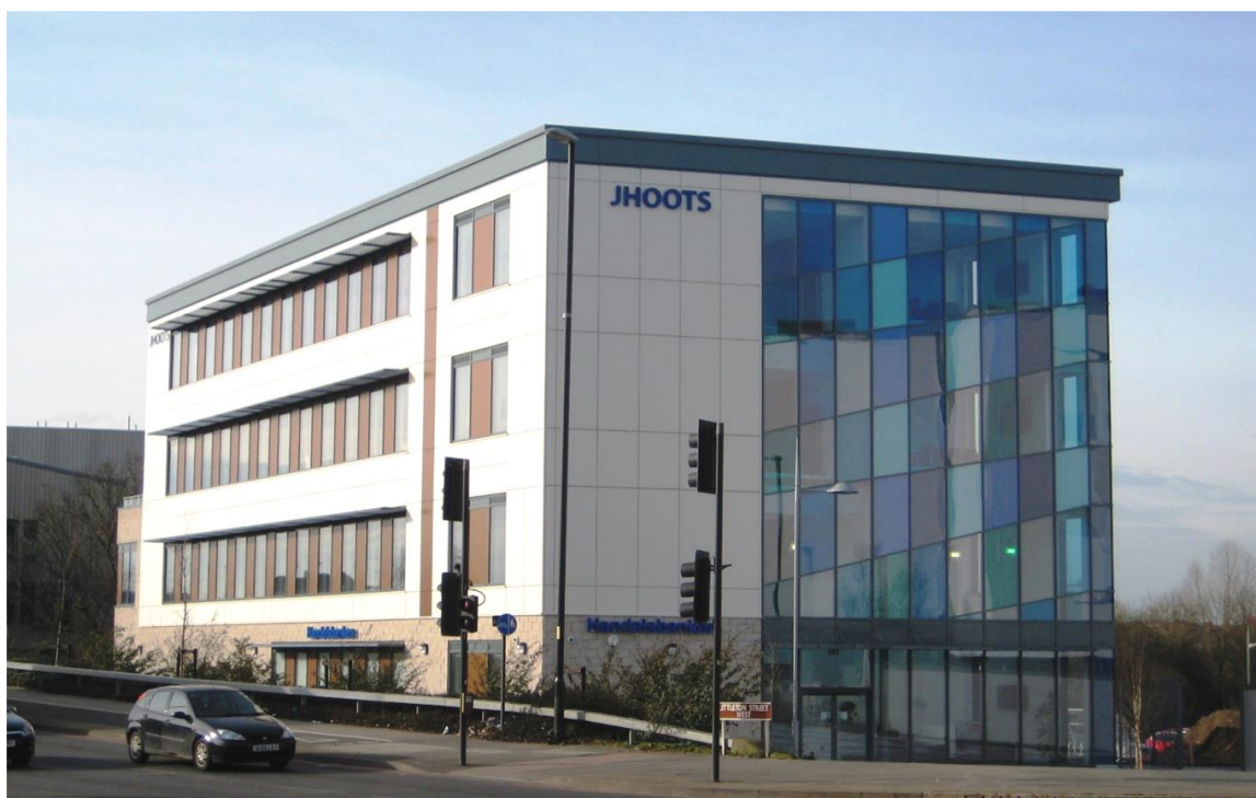
Figure 4.1 Jhoots Pharmacy headquarters, Littleton Street
