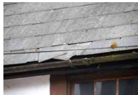
Check for slipped slates
