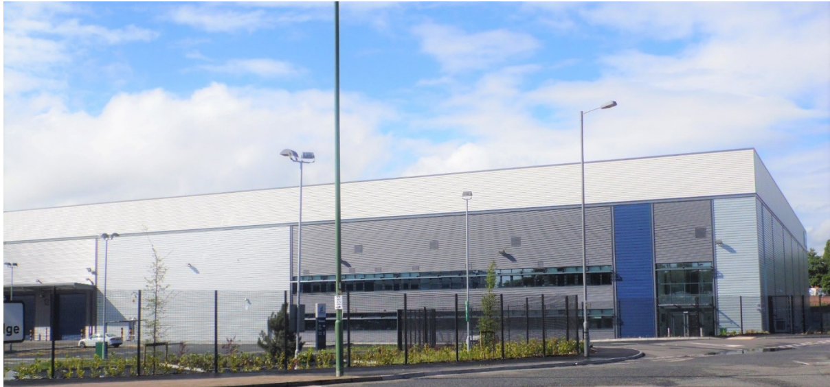
Industrial units at Bull Lane, Moxley completed early 2017
