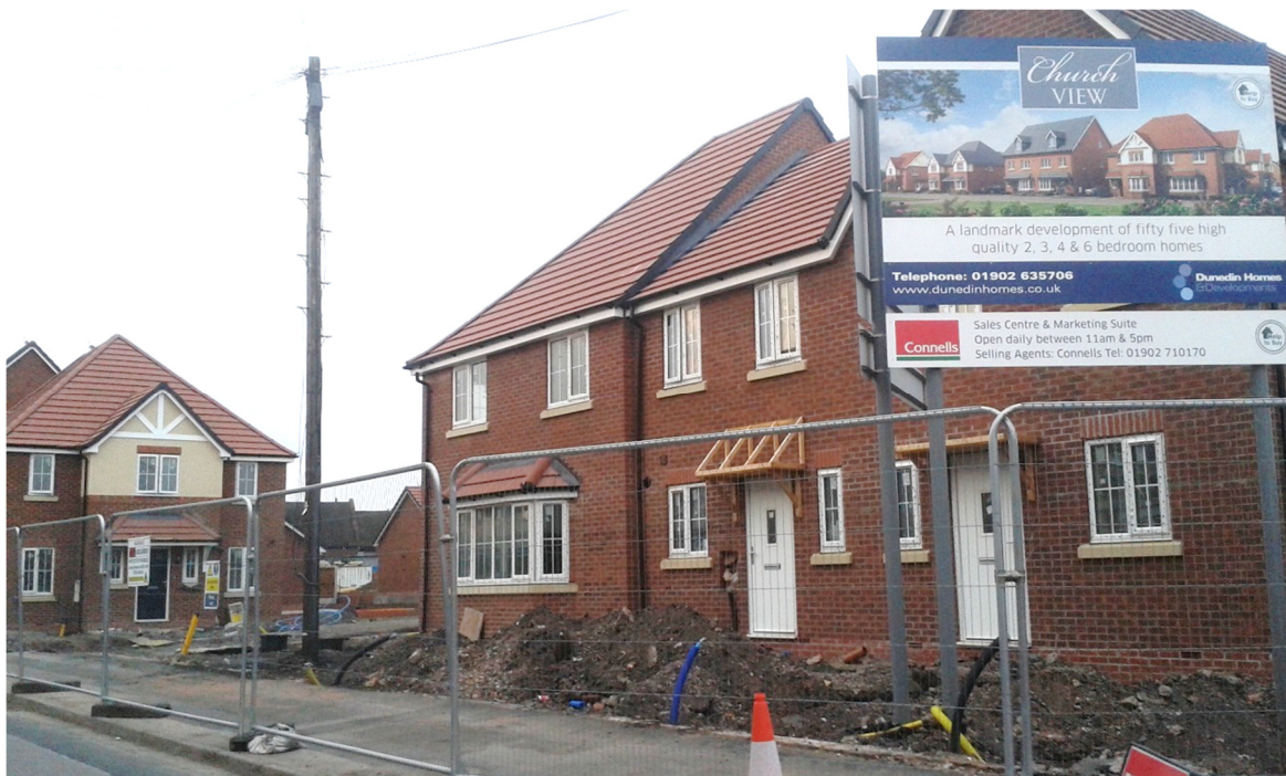
Former ROH Wheels, St Annes Road, Willenhall (August 2015)
