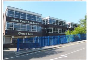
The school buildings are all concrete framed and clad in sections of brown brick with some sections of spandrel panels under principal windows.
