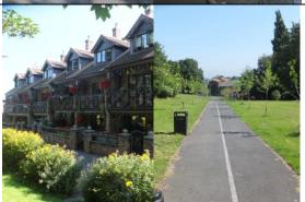
The buildings are all constructed in red brick with some blue brick and reconstituted stone detailing. Roofing is both modern concrete pan tiles and slates and windows and eaves are stained timber. The slow progress of this development has resulted in breeze blocks being a long term external finish across the elevated rear (east facing) elevation of the Hill Street development.
