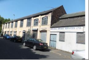
All buildings in the area are constructed in brick and have Welsh slate roofs and cast iron windows. Many of the buildings have been rendered during the 20th century.
