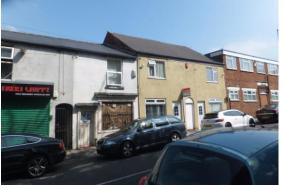
The area is mainly constructed in a semi-hard red brick, dressed in matching moulded brick and roofed in slate. Some buildings have been rendered disrupting the set piece architecture of the terrace or group.
