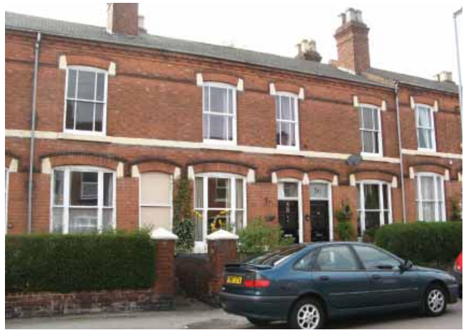
The buildings in Emery Street are covered by the existing Article 4 Direction
