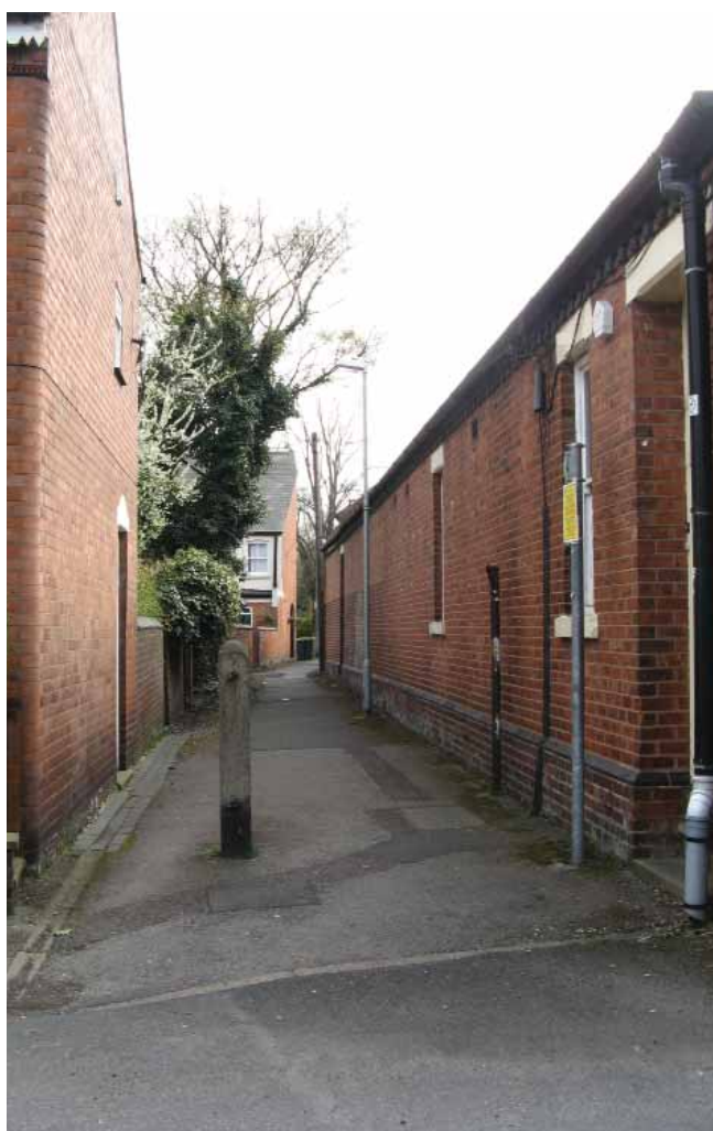
The alley next to Highgate Brewery would benefit from improvements
