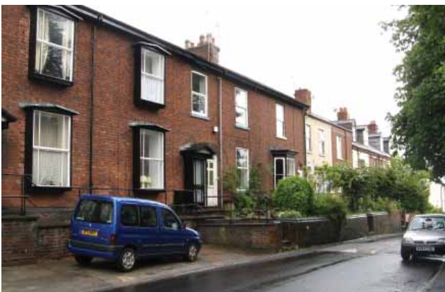
Sandwell Street (north)
