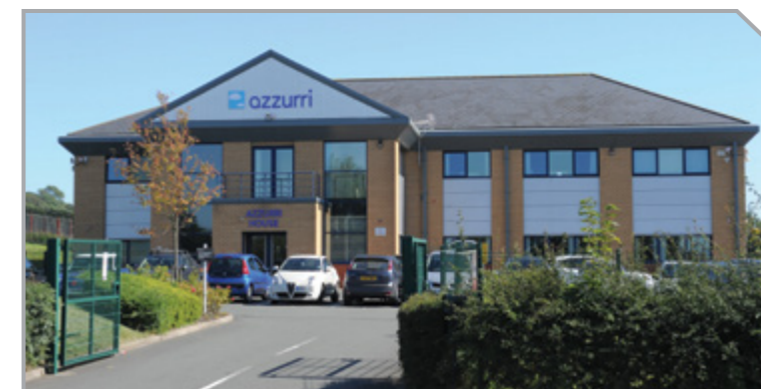
Azzurri House, high quality employment buildings, Aldridge, Walsall
