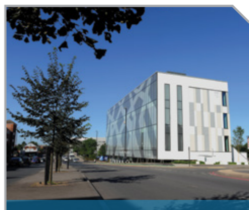
New build offices - Walsall Housing Group
